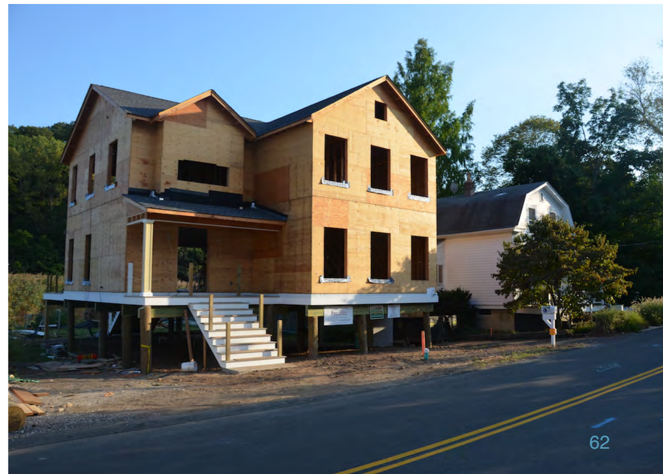
Residence currently under construction in Piermont, elevated on pilings to reduce flood exposure.
