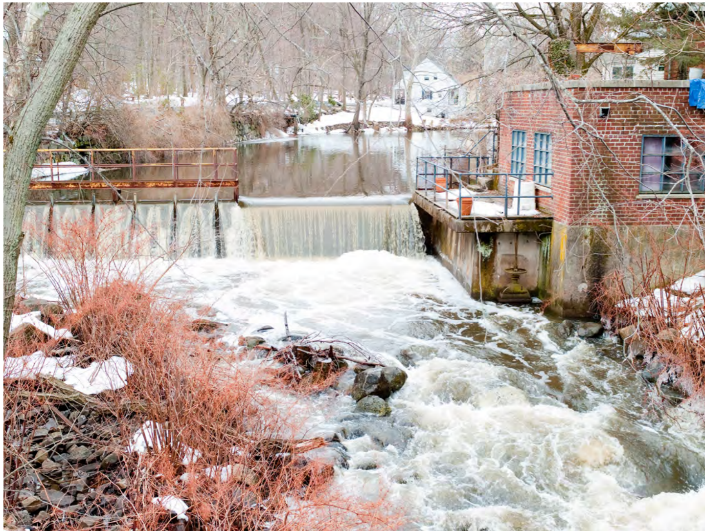
Flooding on the Sparkill Creek.
